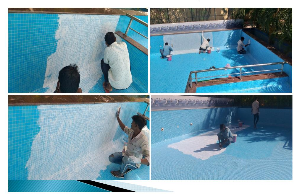
Gap between LED Light & Pool wall Gap filling using Epoxy Grout
