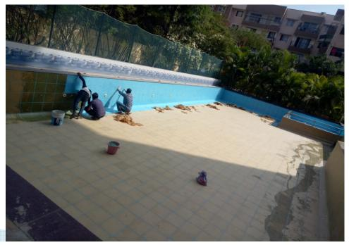
Swimming pool Tiles Epoxy Grouting Work
