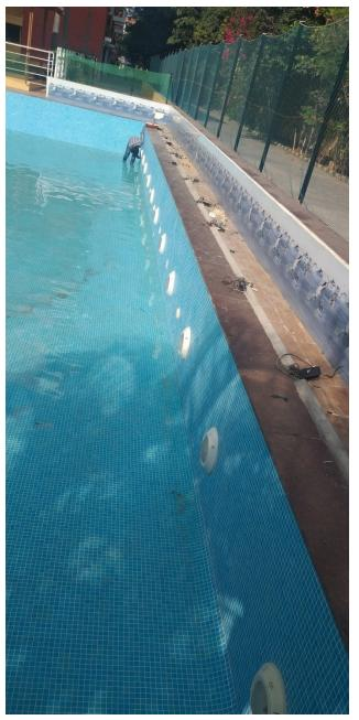
Epoxy Grout filling for Granite joint Gaps.
