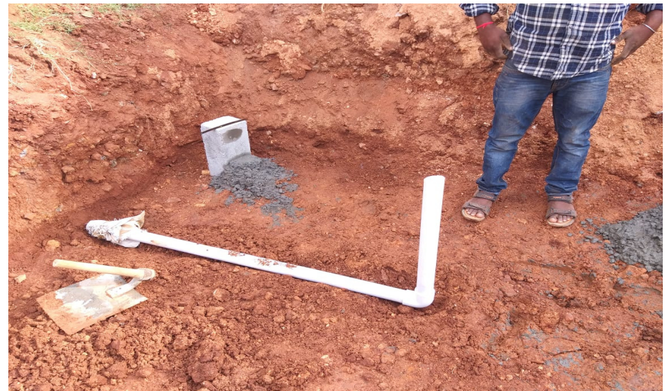
Keeping main drain pipe before floor concrete
