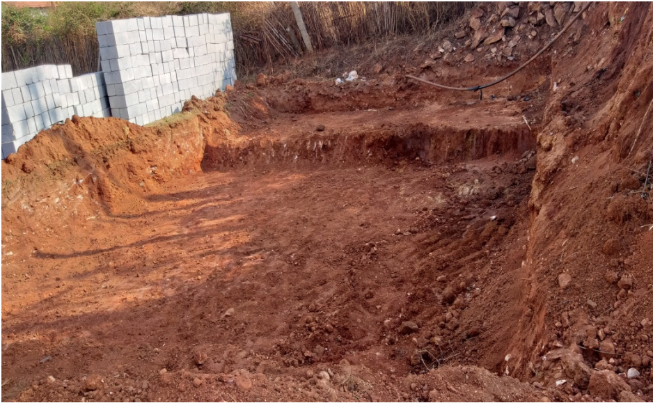
Earth digging for pool construction
