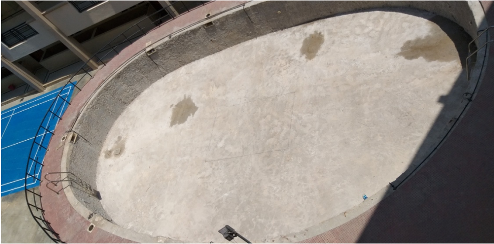
Fully Cleaned & pipelined Pool
