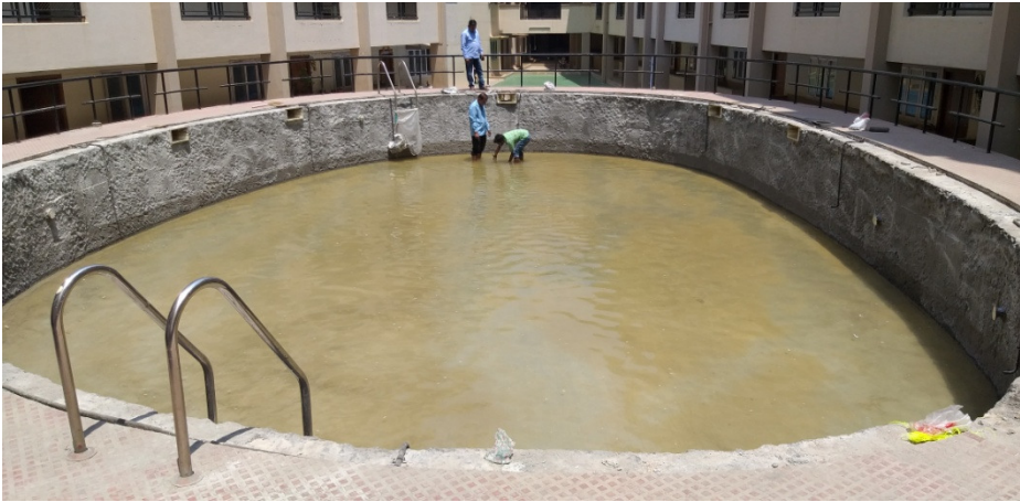
Water filled for Leakage Check
