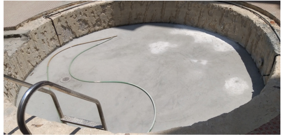
Floor Concrete & Grinding
