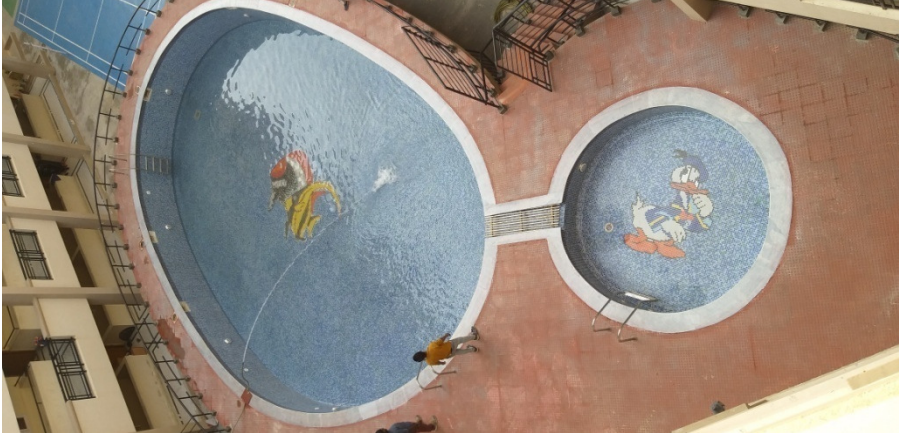
Filling Water To Pool
