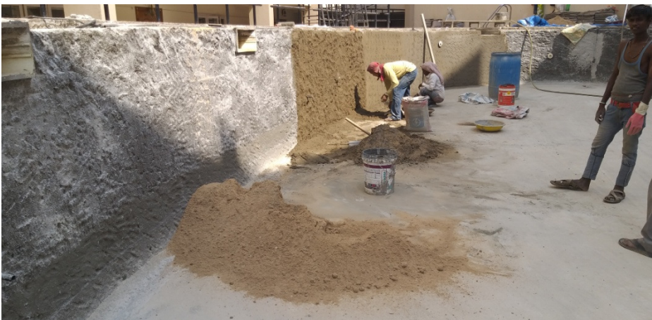
Floor & Wall Plastering
