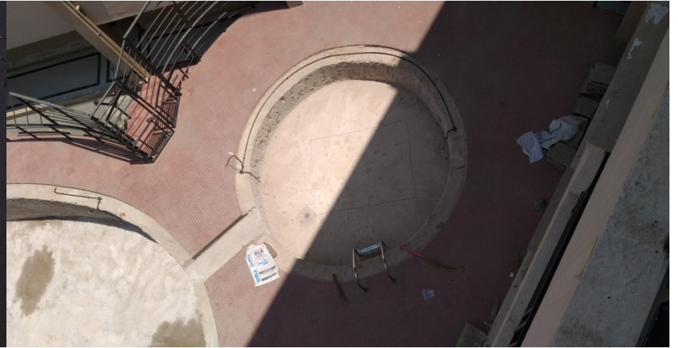
Fully Cleaned Pool
