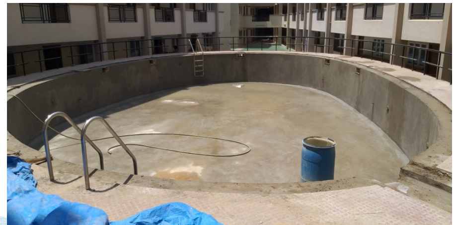
Fully Plastered Pool
