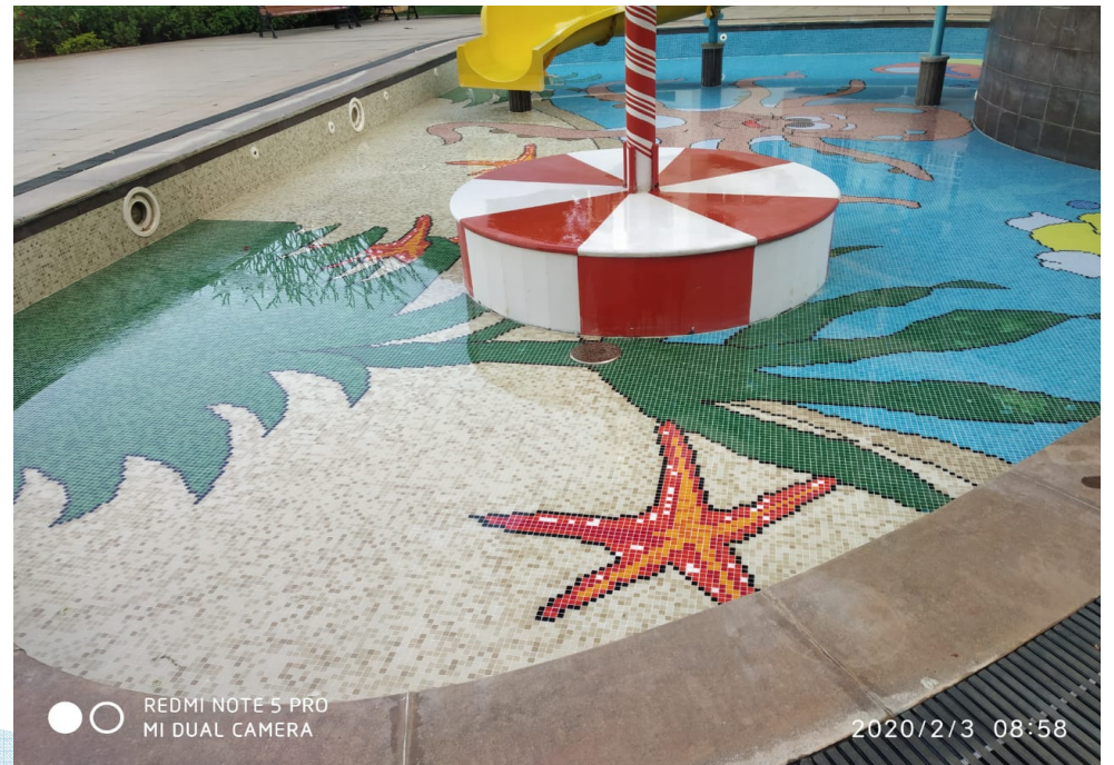
Beautiful View of Main & Kids Pool after Renovation work
