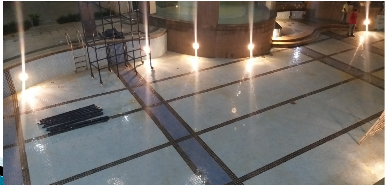
View of Pool with glowing underwater IP68 LED lights
