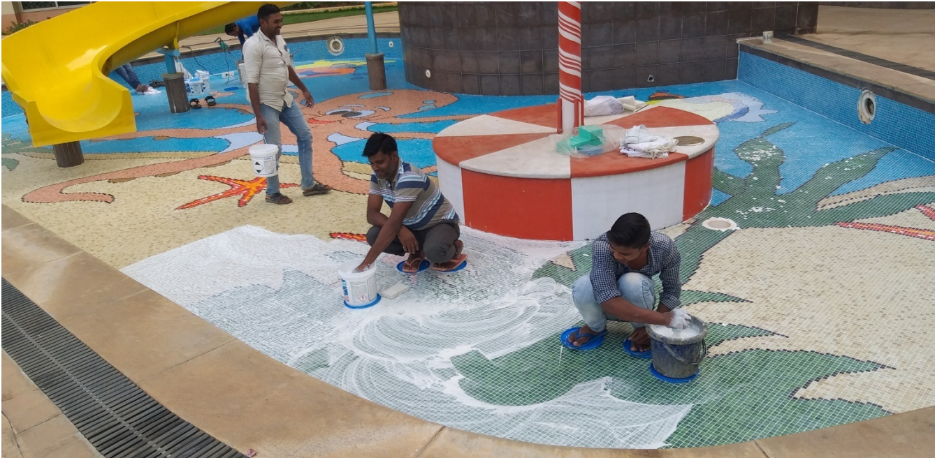
Epoxy Grouting of Kids Pool
