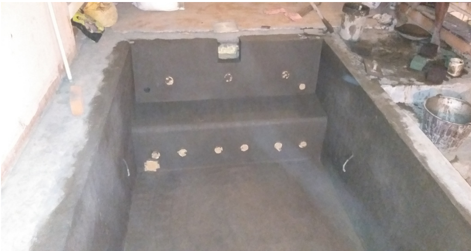
Floor & Wall Plastering
