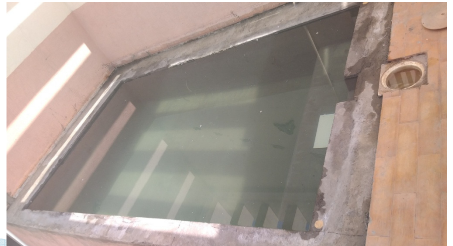
Water Filled for Leakage Check
