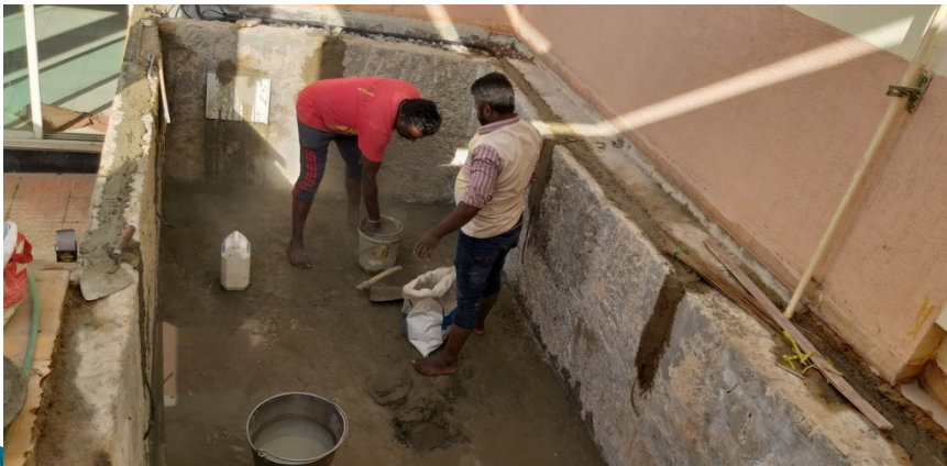
Covering Pipe line & others
