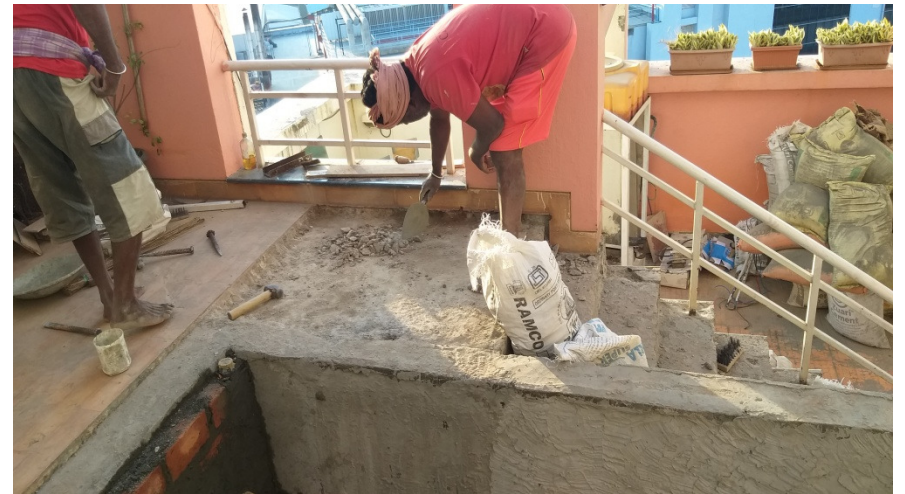
Preparation for Step Granite Fixing
