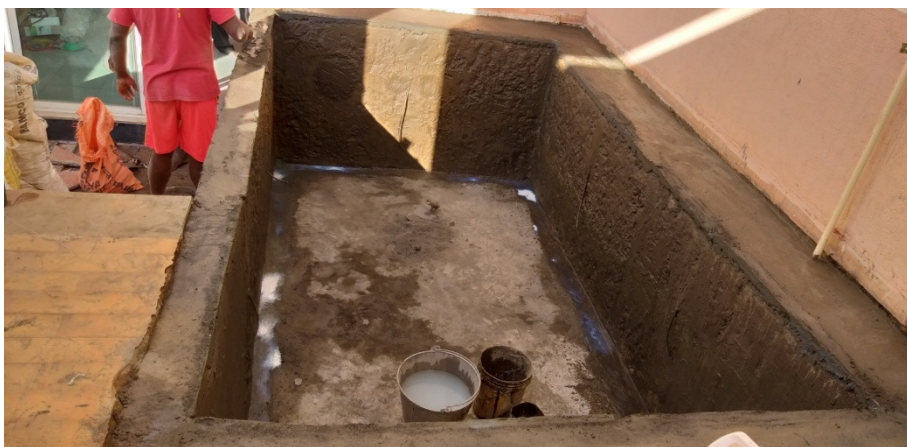
Floor & Wall Waterproofing
