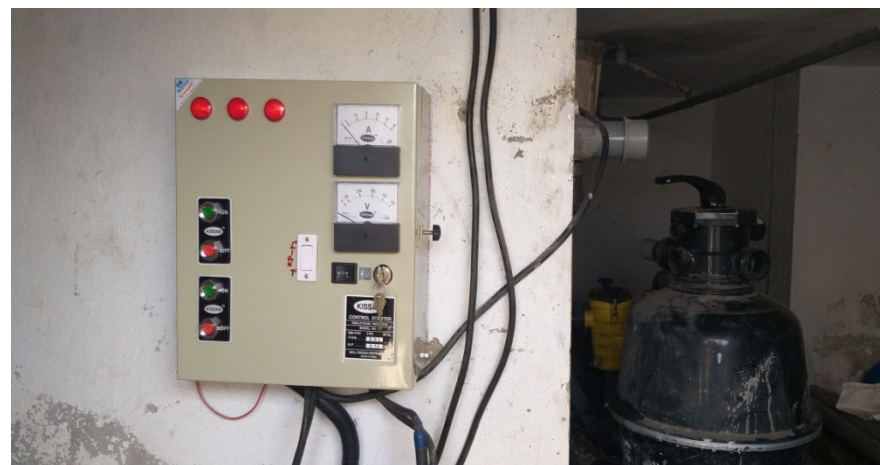
Control Panel for Filtration Room
