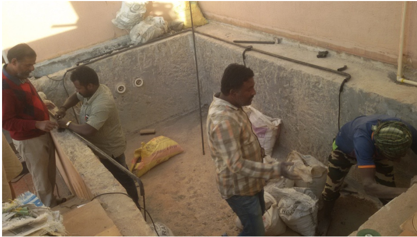
Electrical Pipeline & wiring
