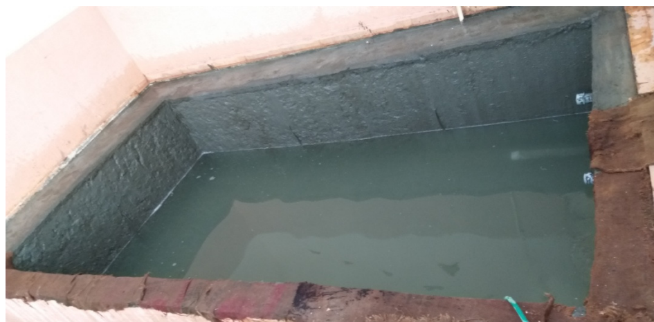
Water filled to check Leakage
