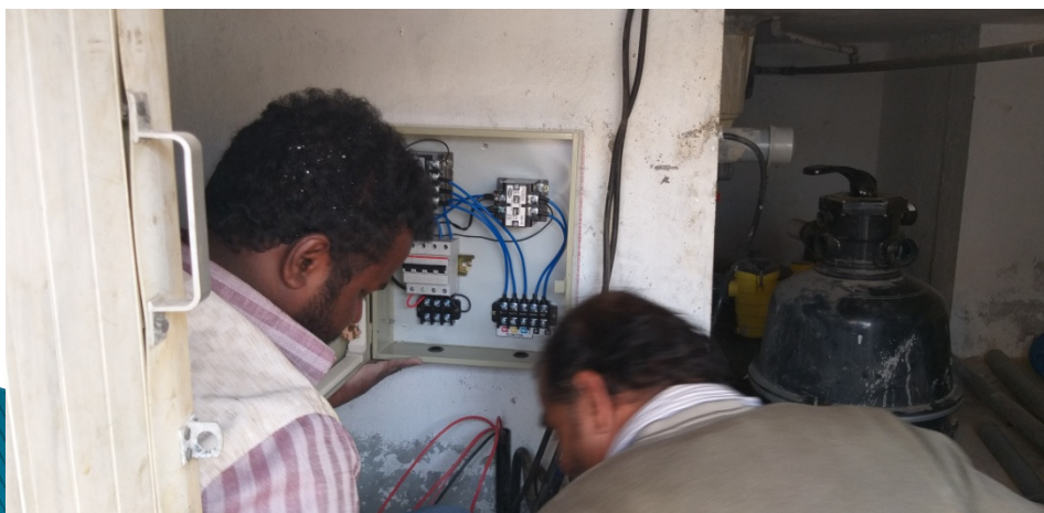
Electrical Control Panel Setup
