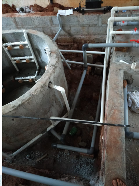
Plumbing work for Filtration system, Connecting heat pump to the Jacuzzi
