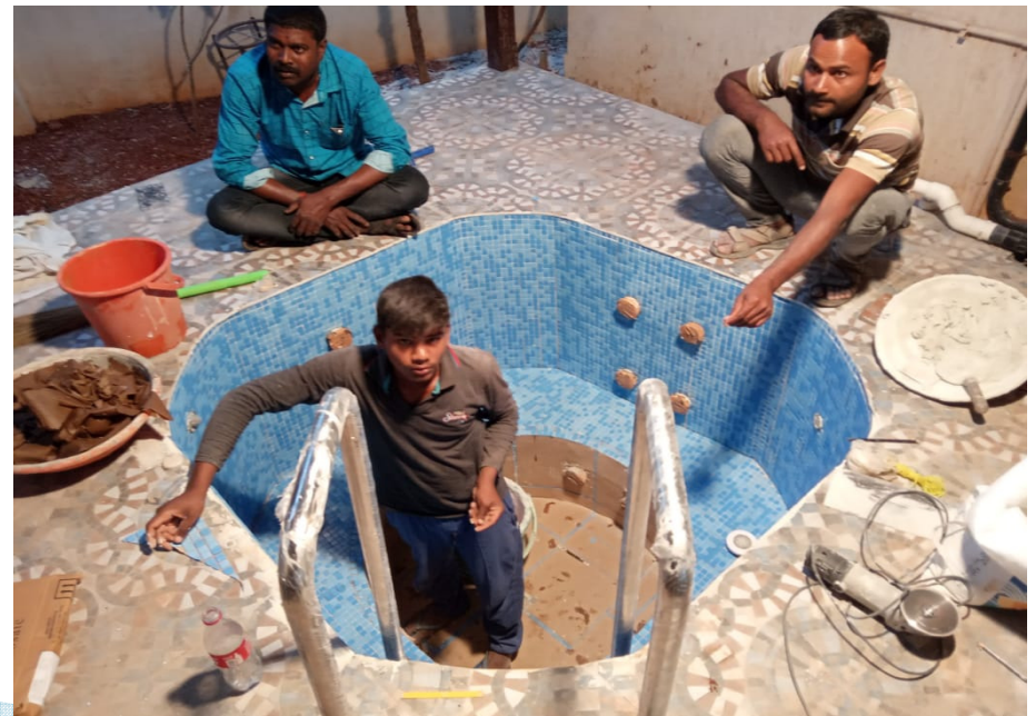
Tile Fixing & Grouting for Jacuzzi Tank
