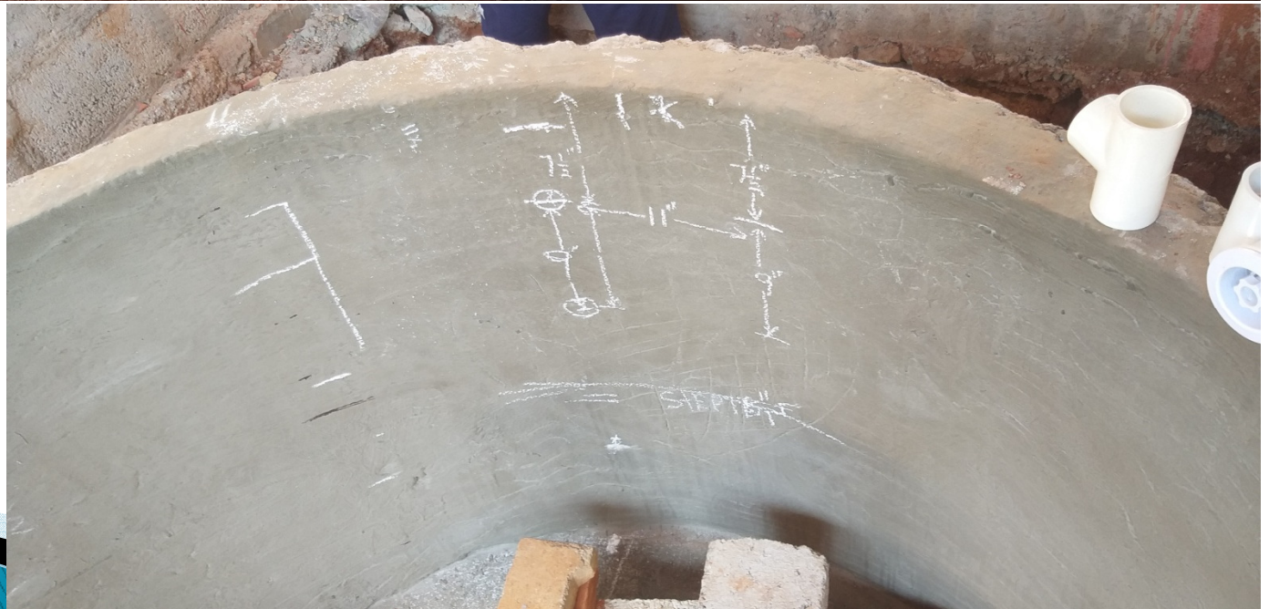
Jacuzzi Tank Construction and Marking for Nozzle setup
