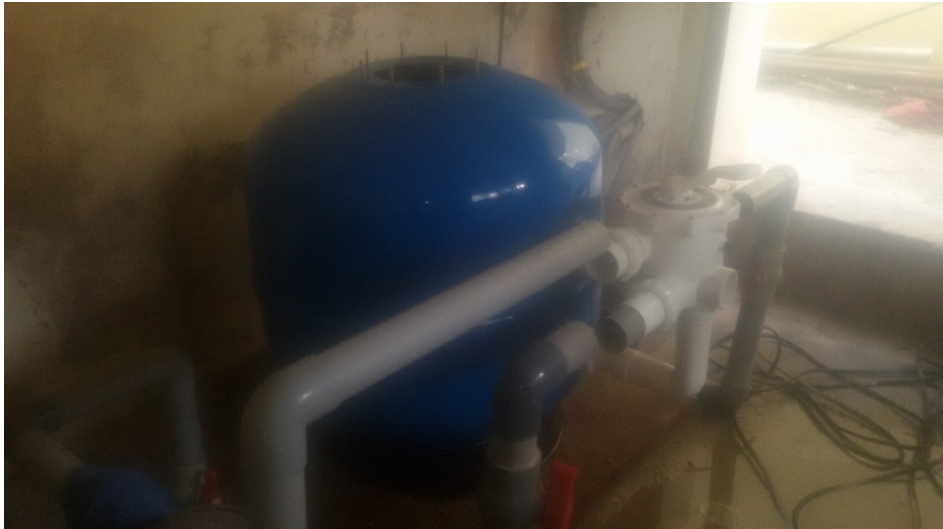
Plumbing work for New Filter
