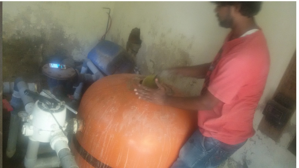
Fixing New Lateral Diffuser Nozzles
