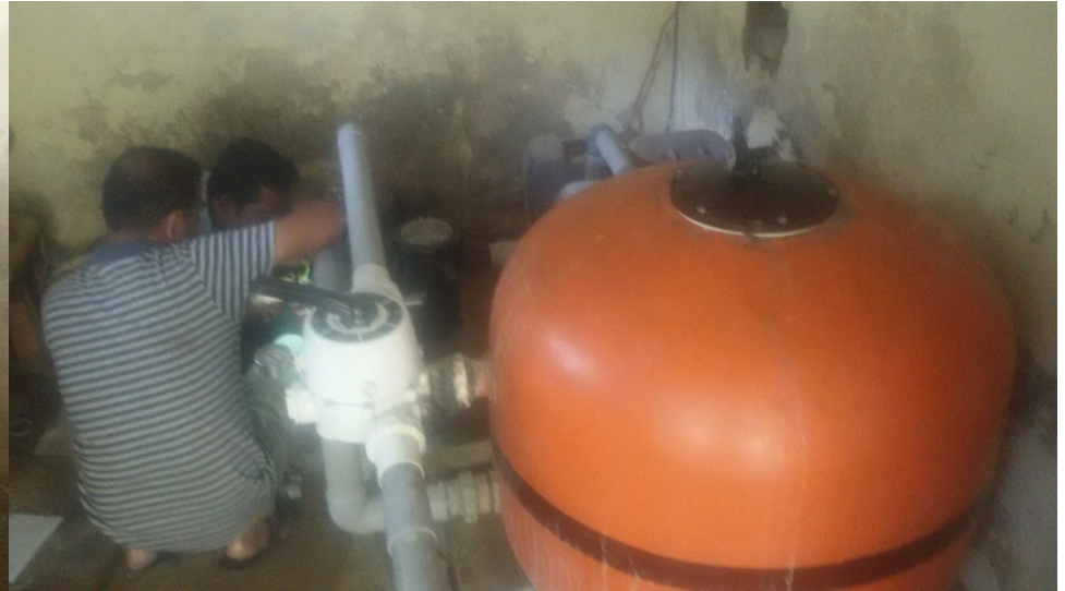
Installation of New Pump
