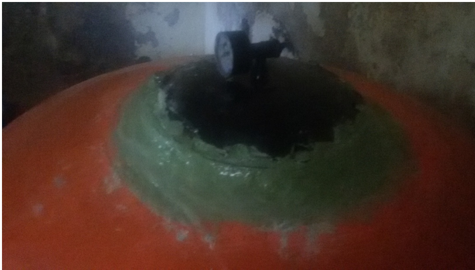
Application of Materials to avoid Leakage
