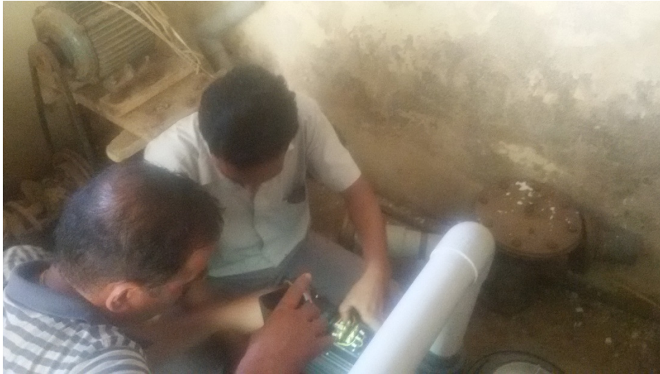
Fixing of New Pump
