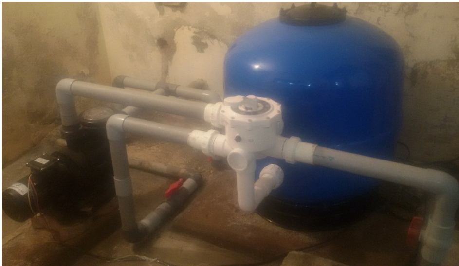
Fixing of valves for plumbing Line
