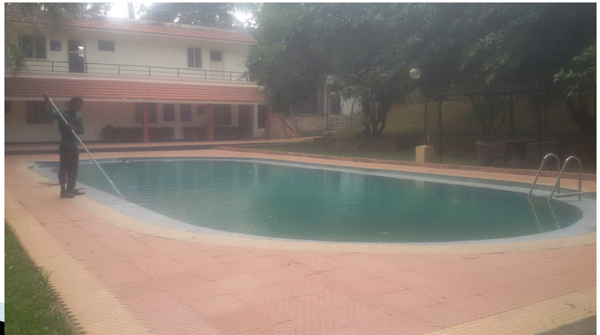
Final view of Pool
