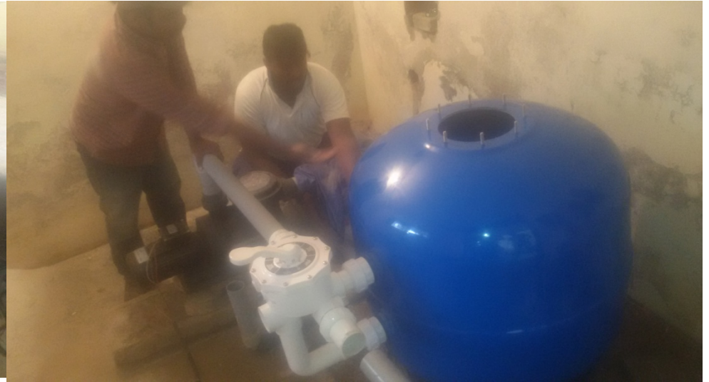
Plumbing work for New Filter
