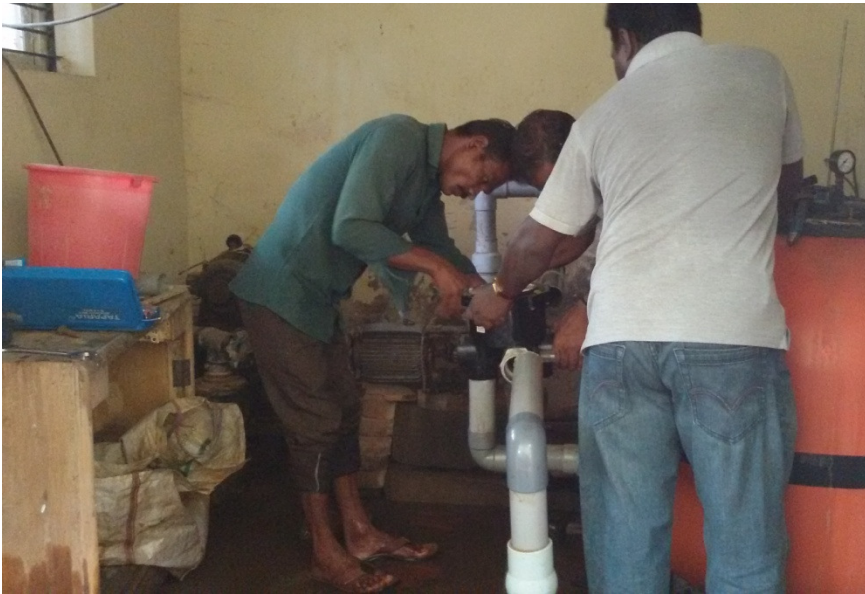
Replacement of Multiport Valve
