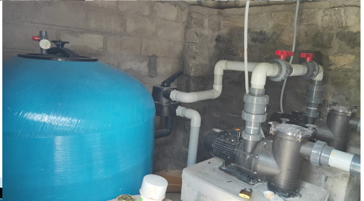
Plumbing Work, Pump & Filter Setup
