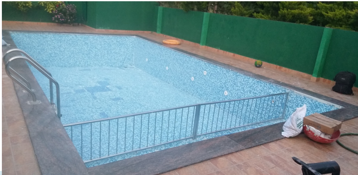
Final View of Pool
