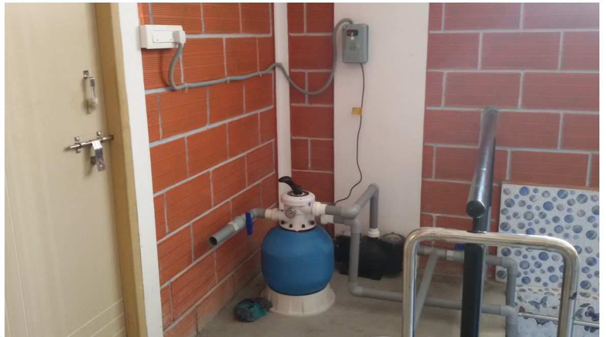
Pool After Filtration setup
