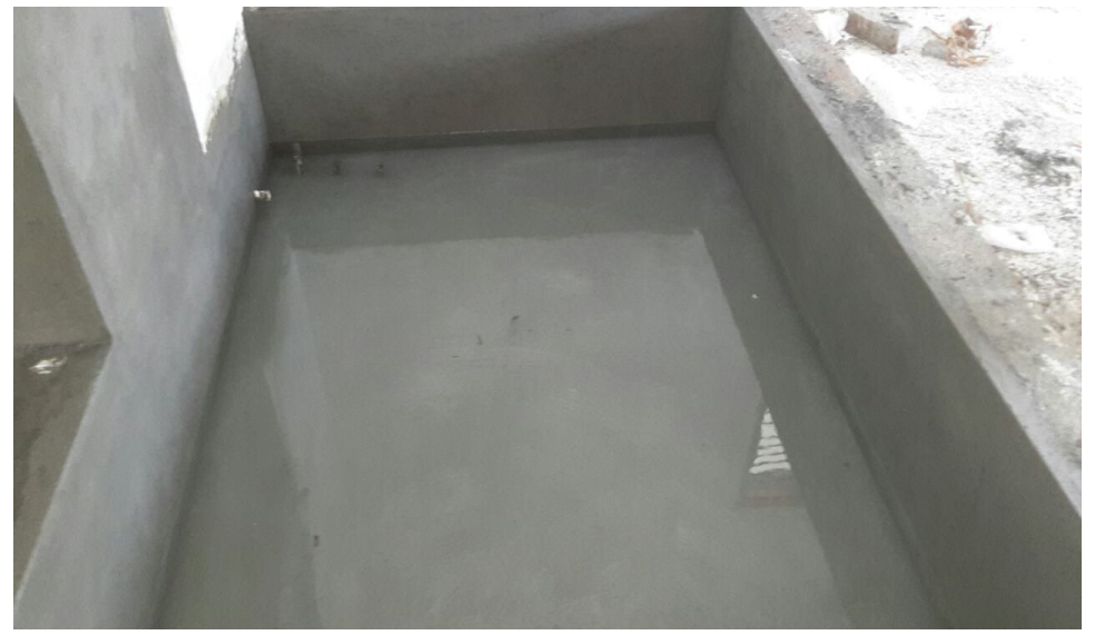
Construction of Balance Tank, Filtration Room & Curing process
