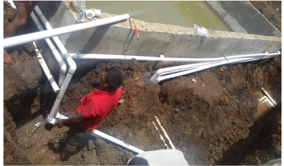
Fixing of Inlet, Suction pipelines, Skimmer Boxes, Filtration Pipeline
