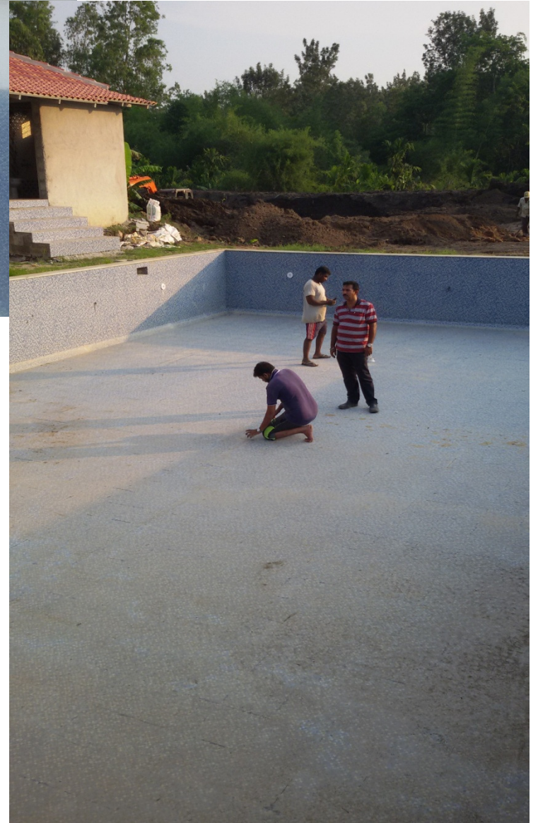
Fixing of Floor & Wall Inlets
