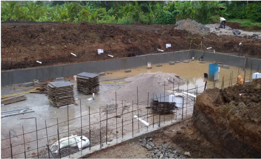
Fixing of Inlet, Suction pipelines, Skimmer Boxes, Filtration Pipeline
