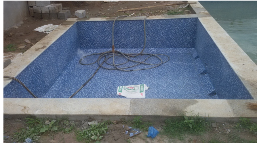
Pool look after Tiling & Grouting Work
